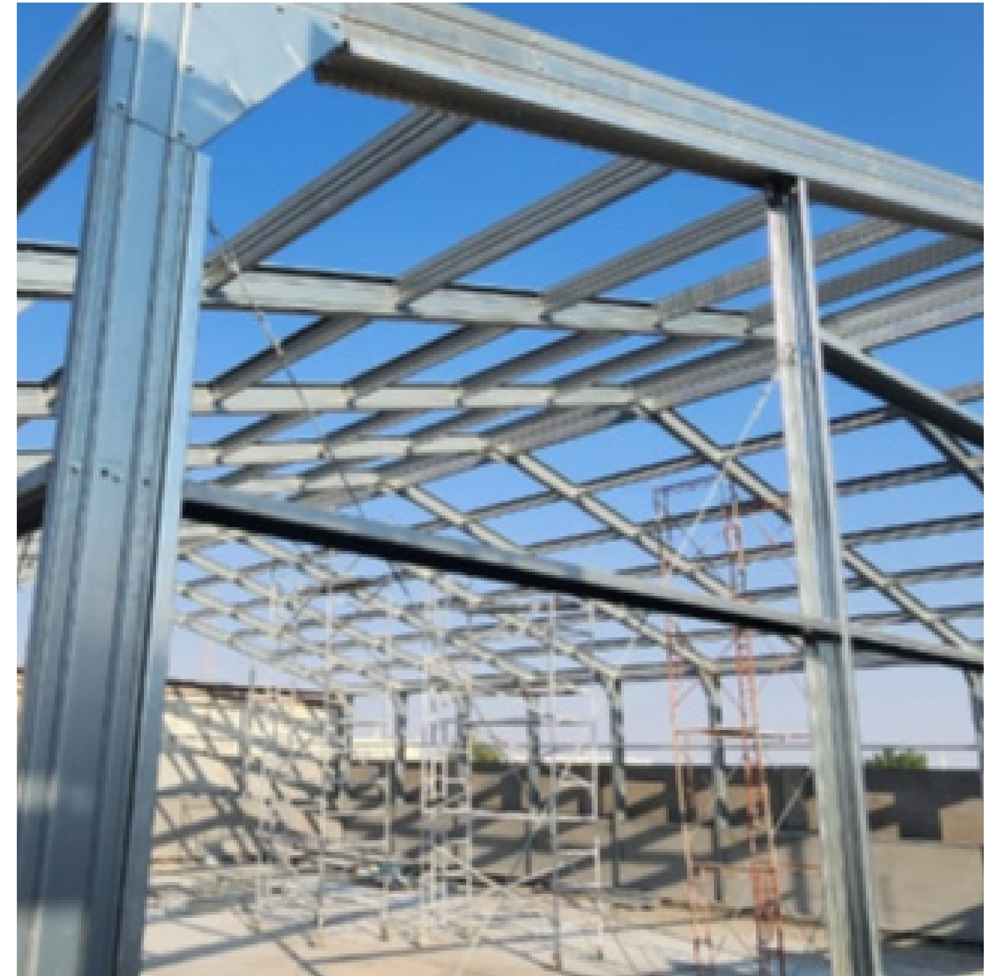
Fabrication and Erection of Steel Storage Hangar – Umm Al Houli
