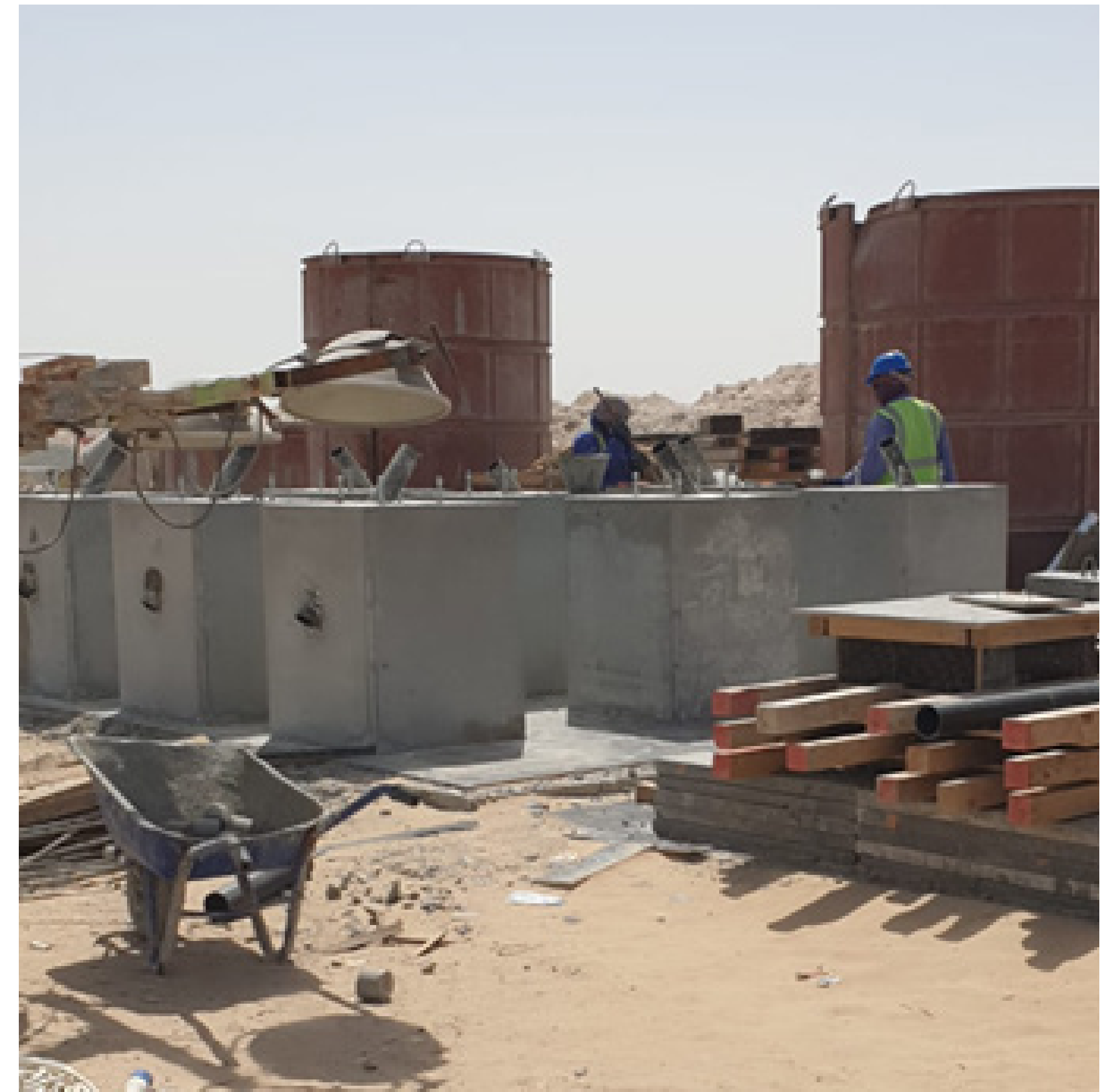
Installation of Solar Powered Lighting Poles including casting of Concrete foundations and battery compartments – Umm Bab Farm Entrances
