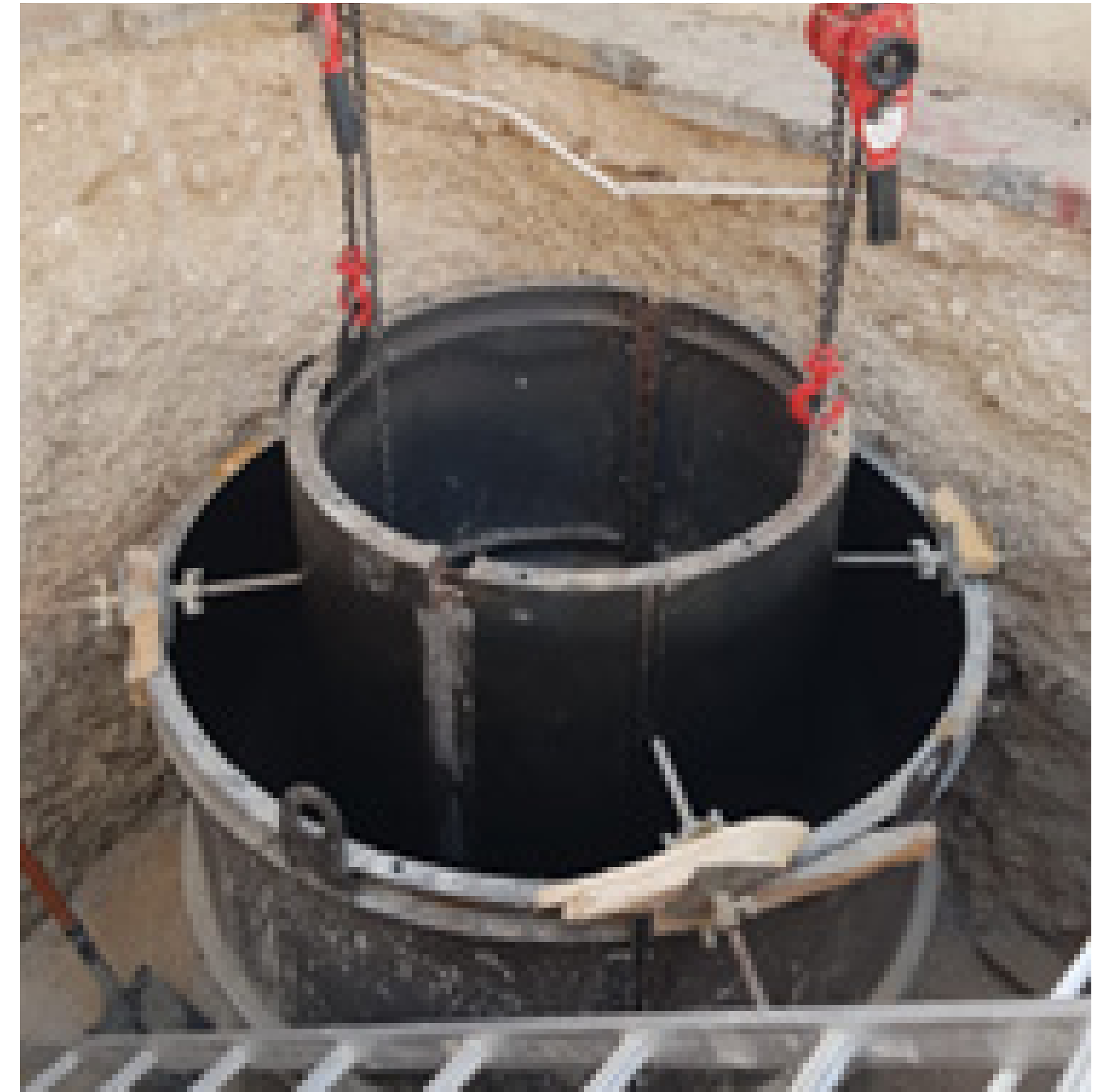
Construction of Concrete Sewerage Manholes for Sewage House Connections
