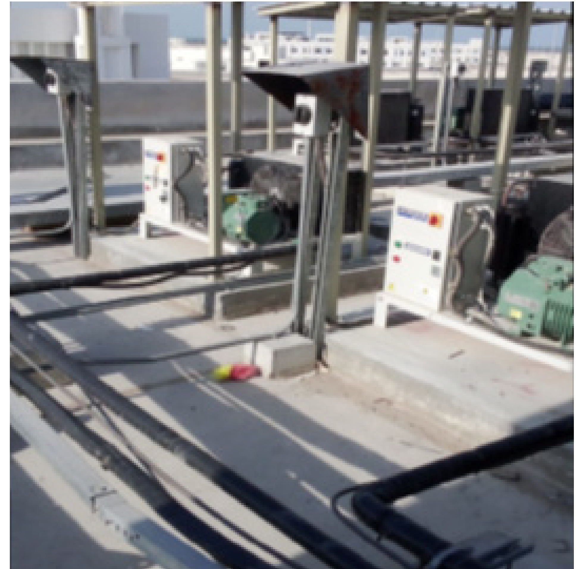
Fabrication and Installation of Roof Shades and Tank Skids
