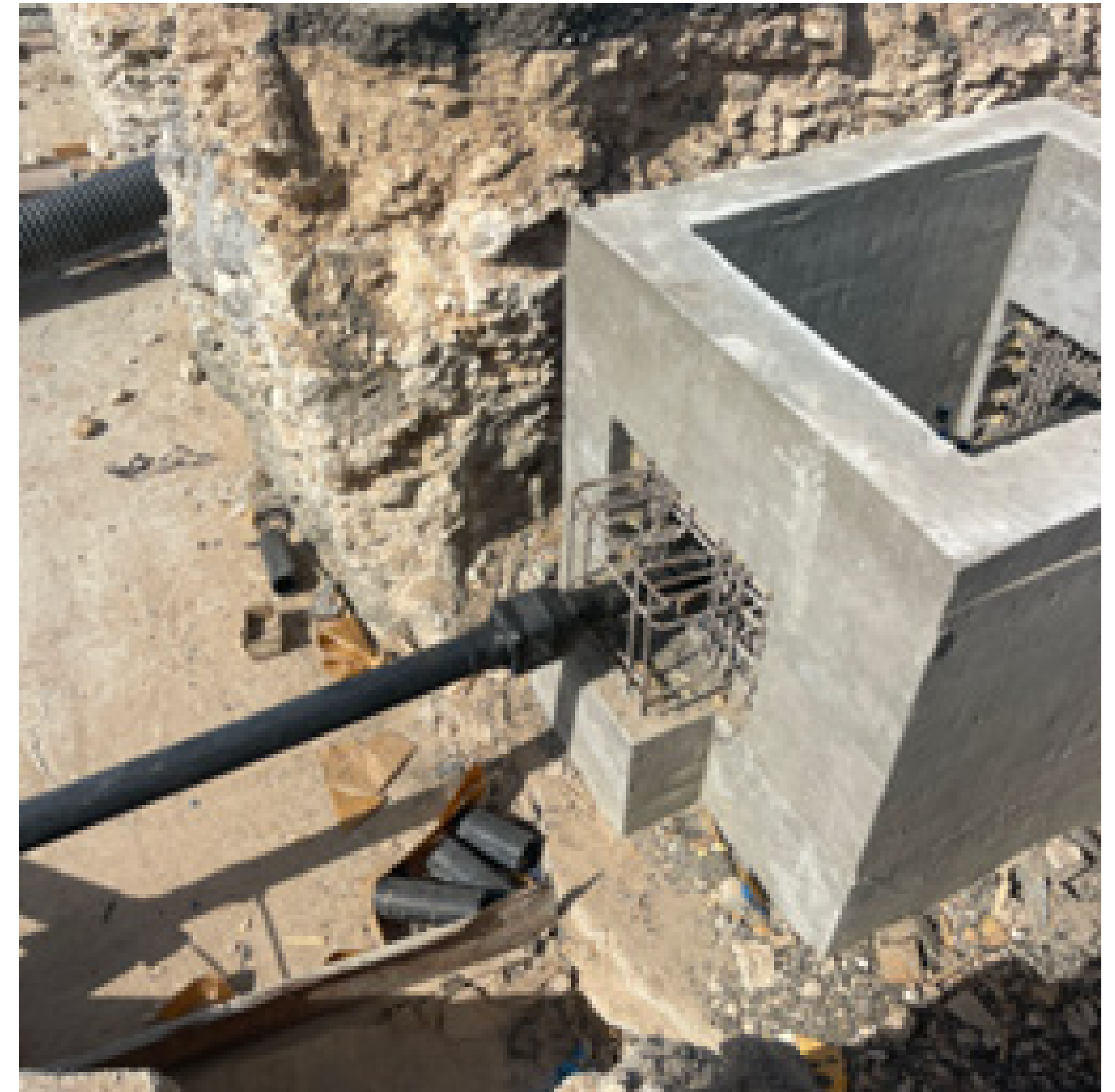
Construction of Underground Valve Chambers and Manholes
